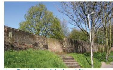
11 Disused pathway into site from Carnoustie Drive
