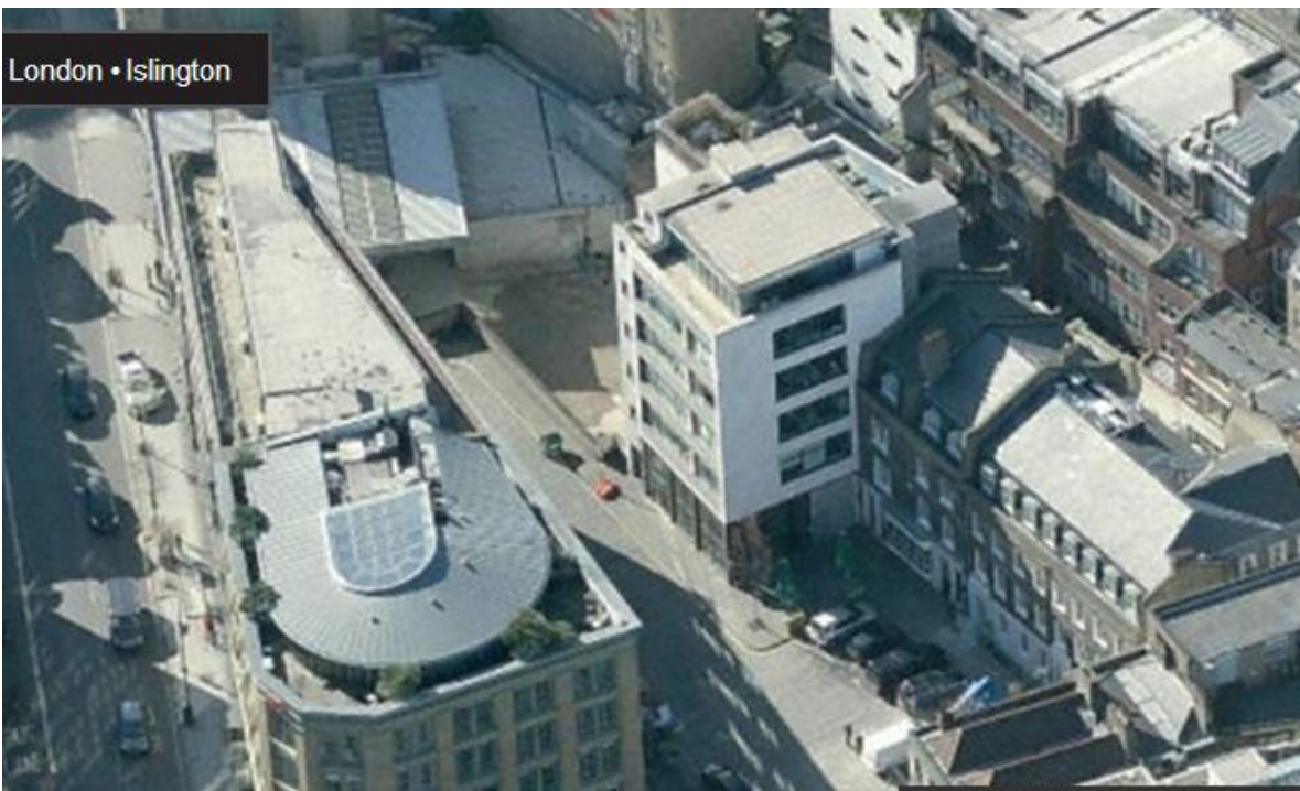
Image 2: Aerial view westwards into the application site from St John's Square.
