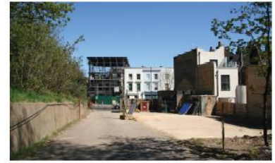
2 Internal access road
