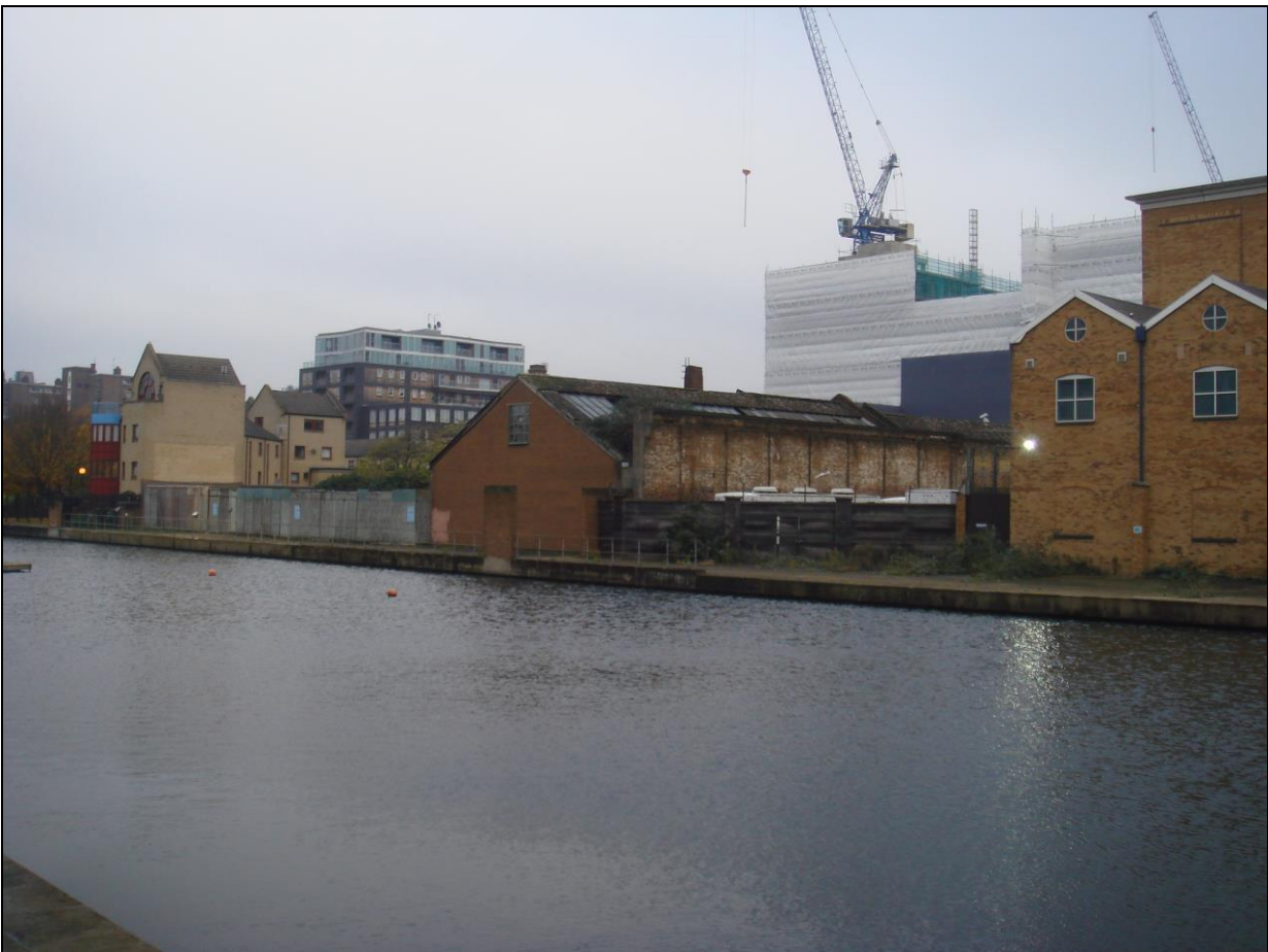
Photograph 3: View from west bank of City Road Basin.
